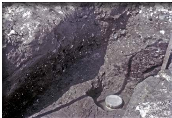
cells 5&6 showing soil sample tin in place
